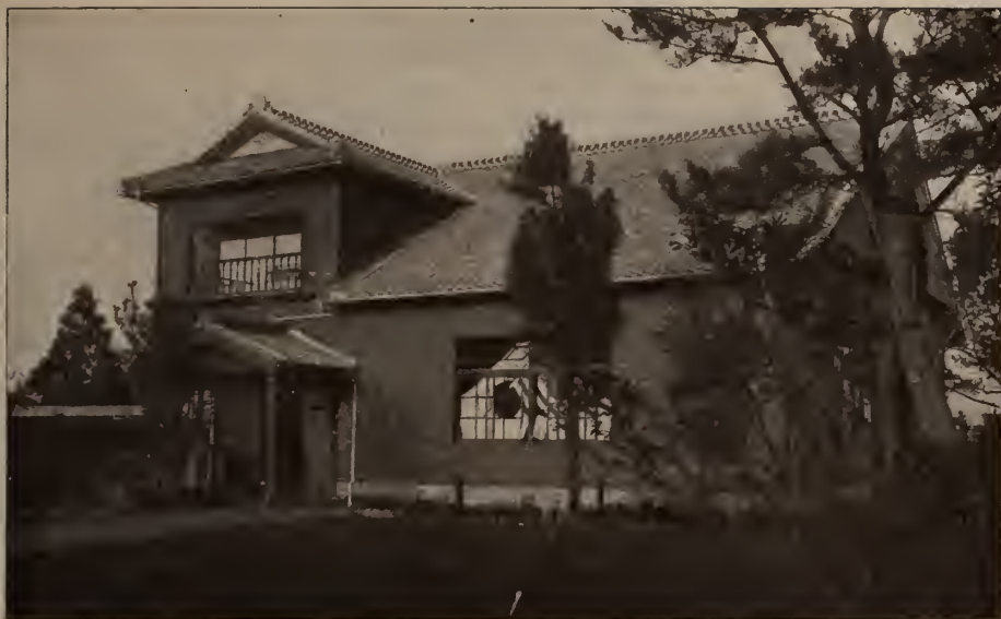
KINDERGARTEN BUILDING AT MIYAZAKI, JAPAN
